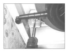
10. Drill out cabinet base through electrical box with 3/4" boring bit.
